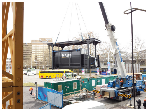
Installation of the hydraulic HABA MEGA system in a ready pit takes only about three to four hours.
