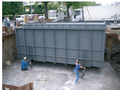
Installation of the hydraulic HABA MEGA system in a ready pit takes only about three to four hours.
